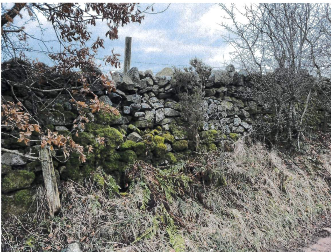
PHOTOGRAPH C – Section of stone bank with wall above then from lonning
